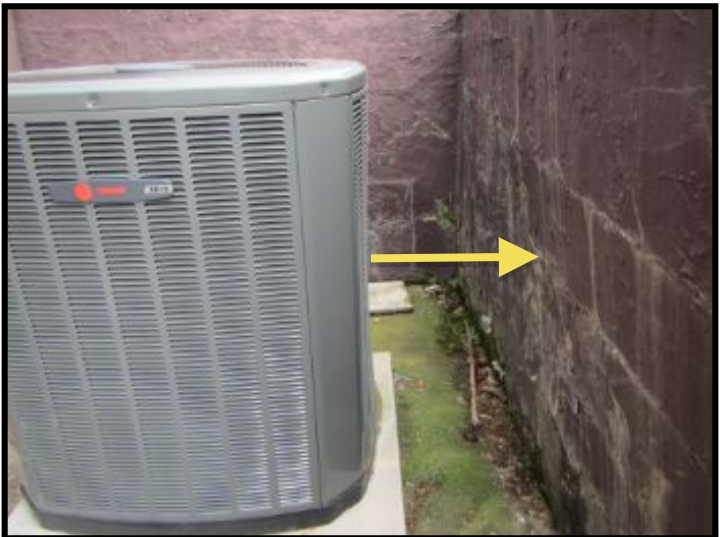
18": The condensing unit was placed within 18" of the structures wall (or other type of restriction: retaining walls, stored items, etc.), this restricts air flow per air conditioner manufacturers recommendations.
