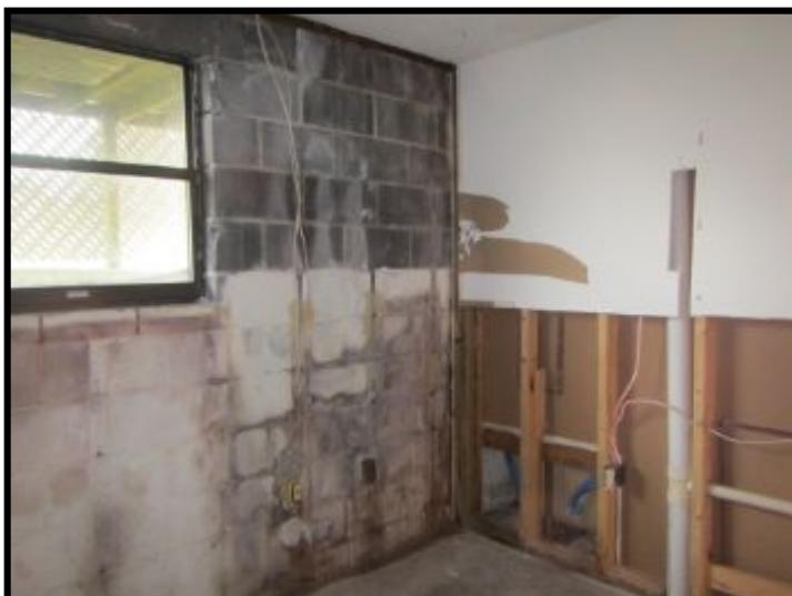
Water stains and Efflorescence on cinder block walls inside the basement. Efflorescence is dried mineral deposits that are transferred from soil/earth by ground moisture through cinder block walls (cinder block being a porous material) on the opposing side of the cinder block wall.
