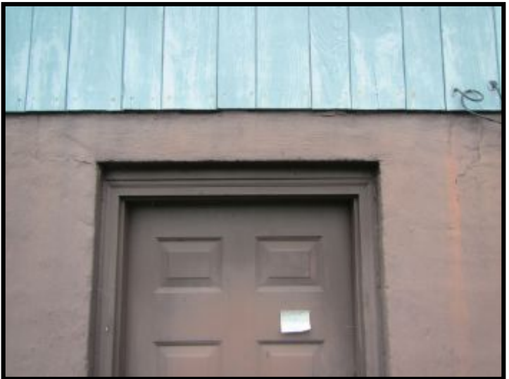
Cracks in cinderblock walls in random areas observed.
