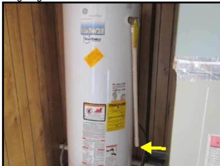
Drain line was too short from the temperature pressure relief valve
