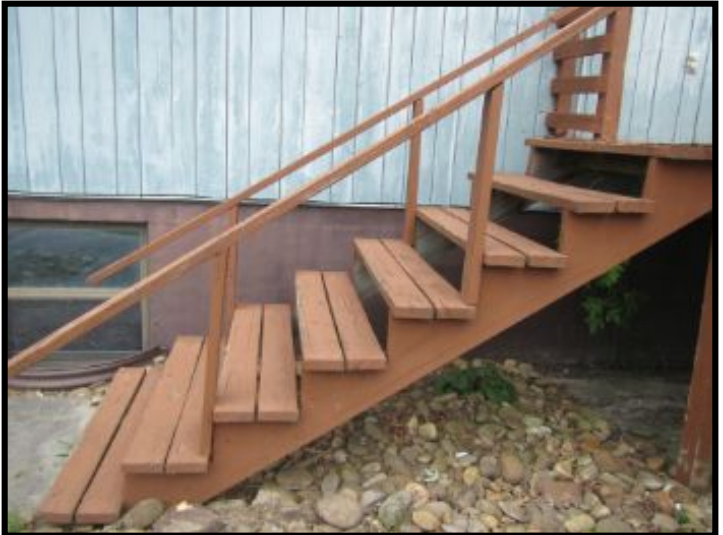
The handrail to the step case was below today's industry standard height and balusters were missing from the handrail.
