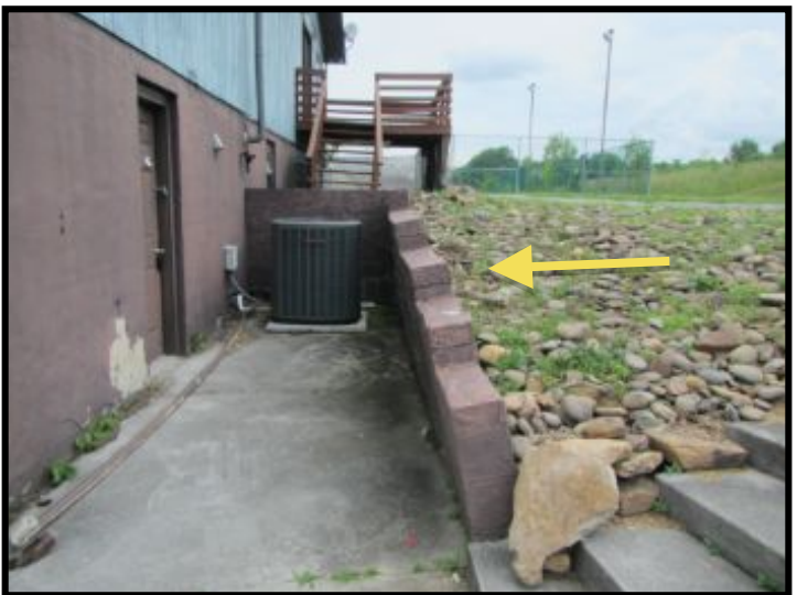
The retaining wall was leaning at the back of the structure.
