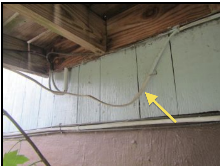
Electrical wiring below the back deck was not protected in electrical conduit.
