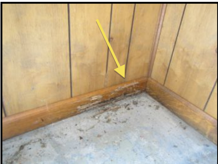
There was wood decay on the baseboards at the front right corner in the garage.
