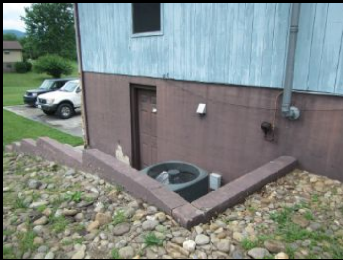
A guard rail should be installed at the top of the retaining wall when the grade differentials are greater than 30" apart per today's International Residential Code building practices.
