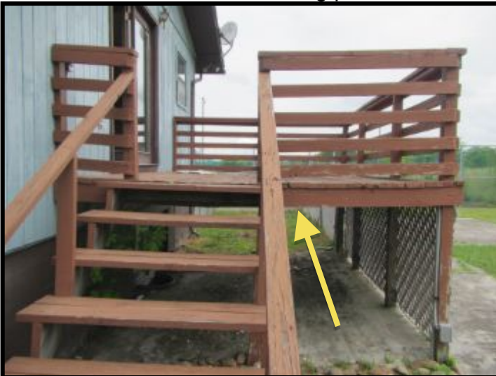
The back deck's joist sagged in the middle/walking surface sagged.
