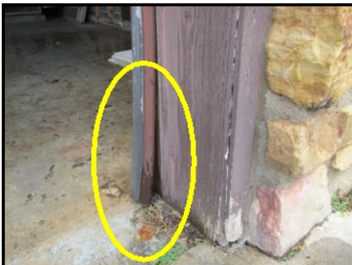
weather strips were insecure at the garage overhead door
