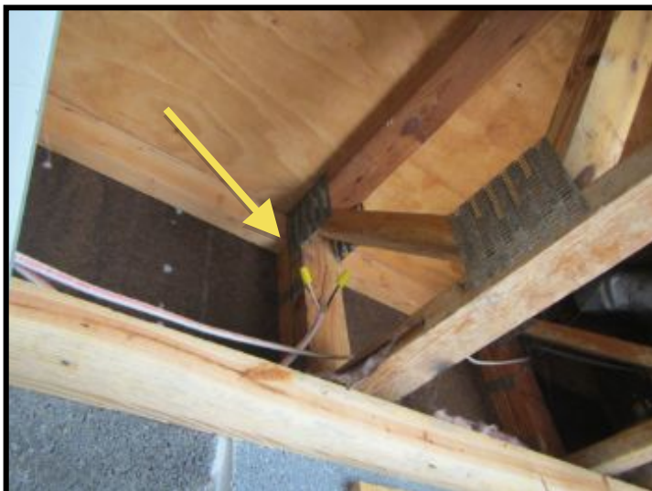
Wire ends not in junction box in garage above back exterior door.
