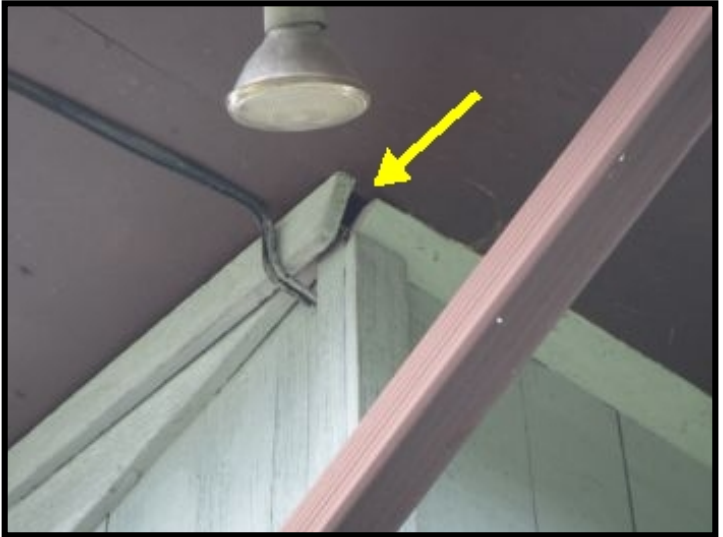
Frieze board was separated and appeared insecure at the back left corner under the eave.
