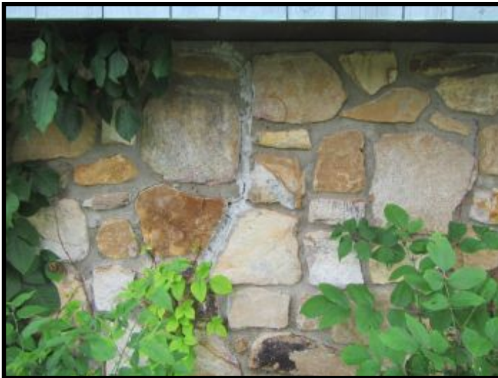
Some hairline separation between the stone siding and mortar in random areas observed.
