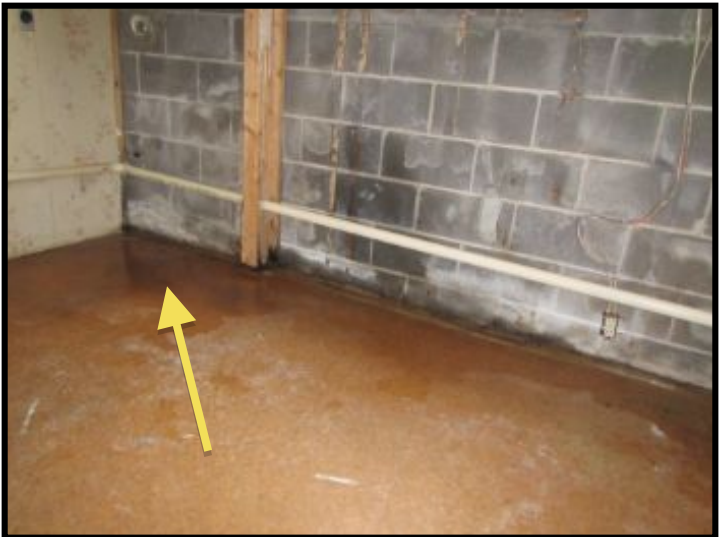
There was water on the floor in the basement utility room at the time of the inspection.
