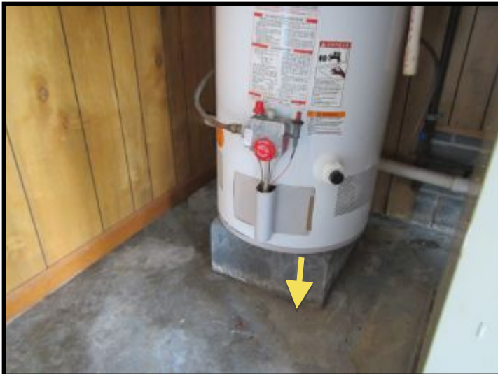
Unit was not elevated 18" as required when unit is located in the garage
