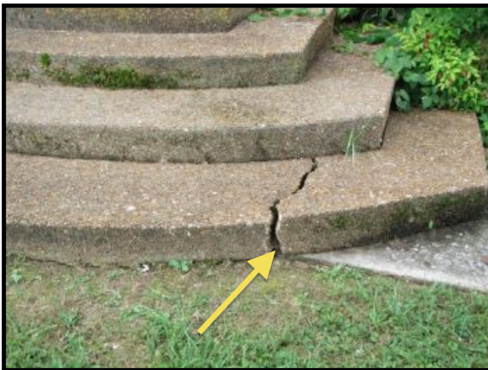
The front porch steps were cracked.
