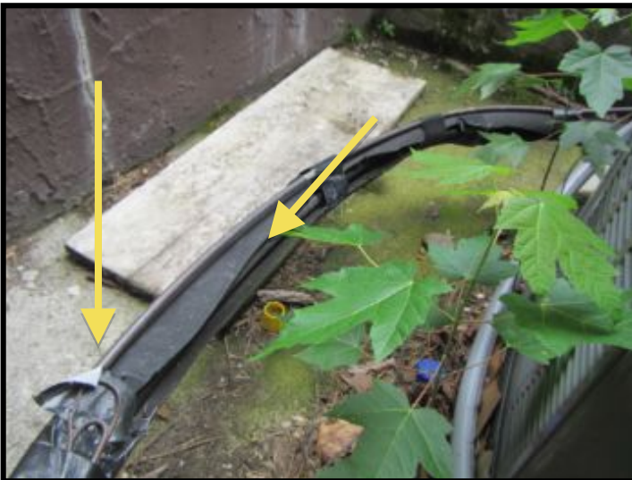
Insulation was damaged/missing at copper tubing connected to the condensing unit
