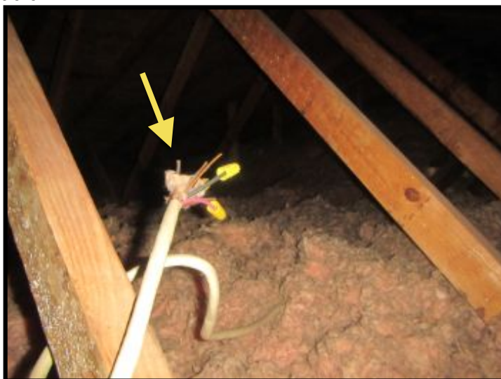
There was an unterminated wire end in the attic at the access.
