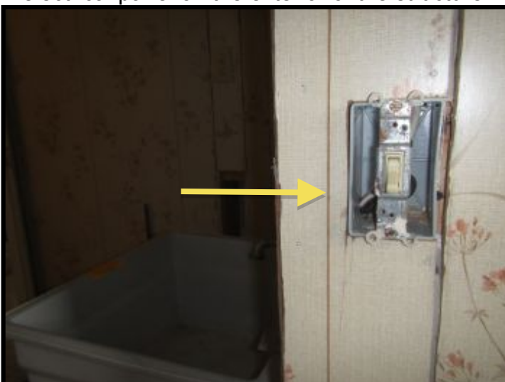
Missing outlet and/or switch coverings in random areas throughout structure
