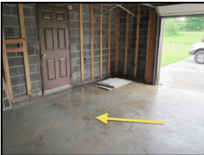
water on the floor in the garage at the time of the inspection
