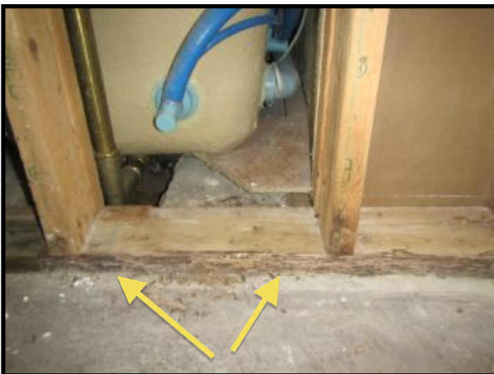
wood rot on sill board behind basement bathtub
