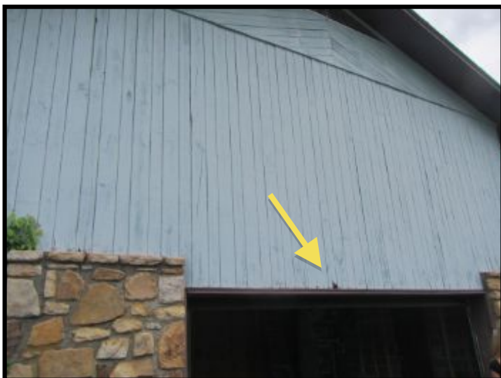
There was wood rot on exterior wood siding at more than one location, including trim around windows and doors.
