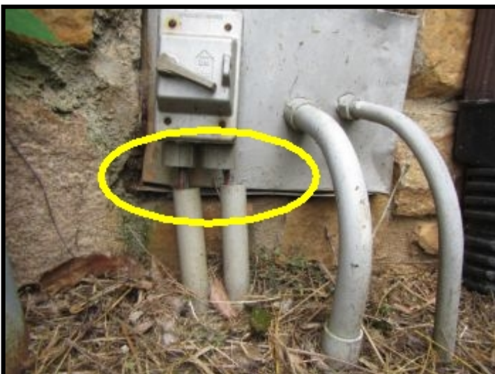
Conduit was insecure at branch wiring below the electrical panel on the exterior of the structure.
