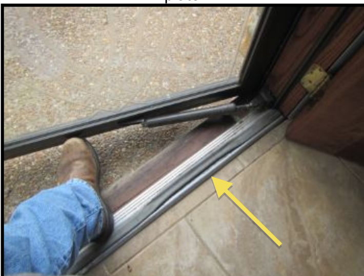
The seal was damaged at the front door threshold.
