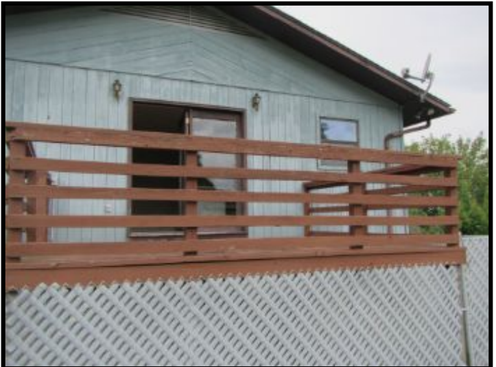
Wood rot on multiple members of the back deck. Fasteners were backing out at several locations.
