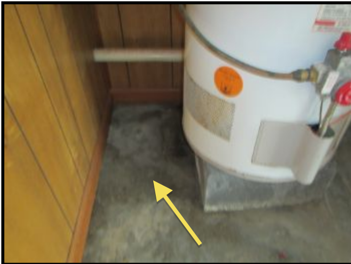
Note that there were dry water stains on the floor below the water heating unit in the garage.
