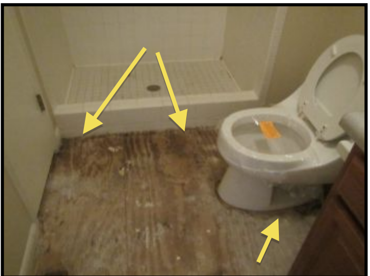
Note that there were dry water stains on the floor of the master bathroom.
