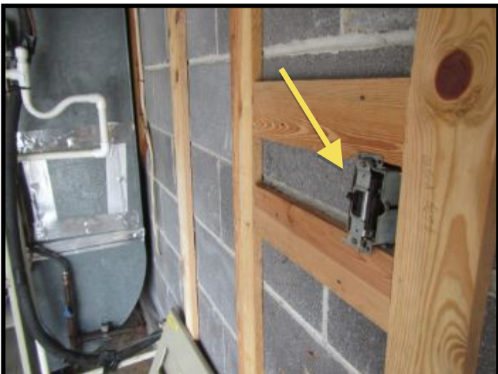
The switch on the back wall in the garage was missing a cover.
