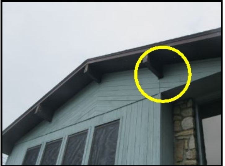
Trim was insecure at the right side beam protruding out from the exterior wall at the front of the living room.
