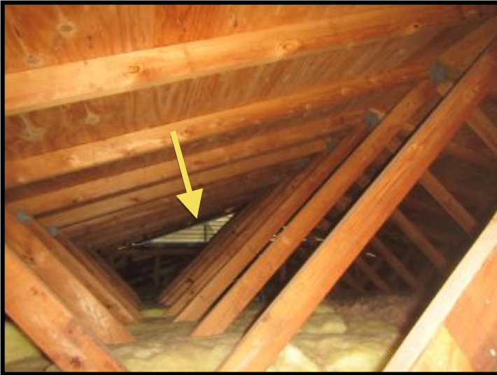
Screen was damaged at the gable vents.
