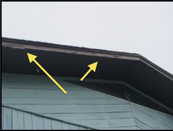
The rake boards had damage at the right side above the garage access wall.
