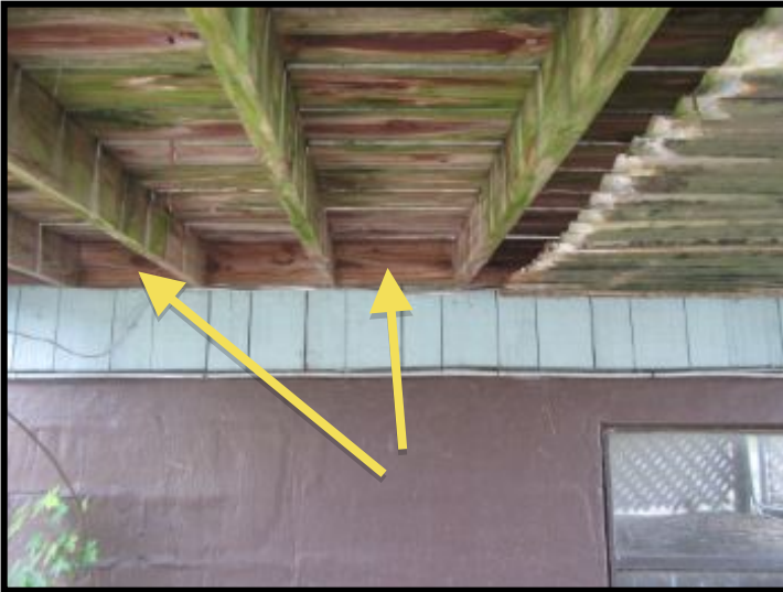
Deck was not lag bolted to the structure.
