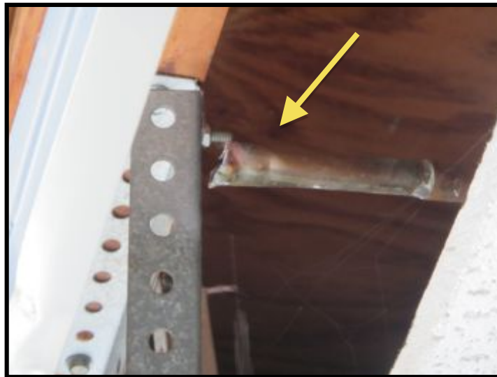
cut copper water pipe in ceiling of garage
