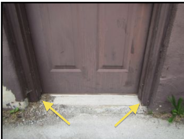
There was minor wood rot on the exterior frame/trim boards at ground level at the back exterior walk through door from the garage. The door did not close and latch in the frame/strike plate.
