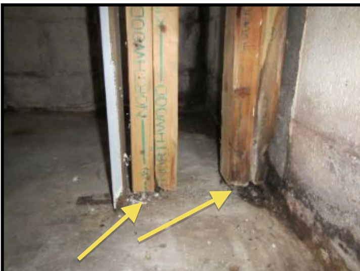
Sill boards were missing at walls in the basement.
