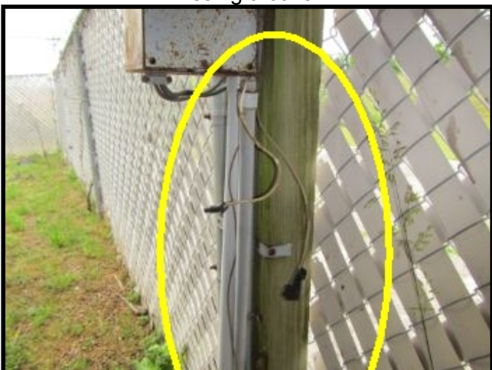
There were improperly terminated wire ends coming from conduit below the back left corner of the back deck.
