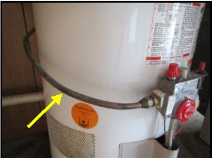
Copper tubing was in use as gas supply line.
