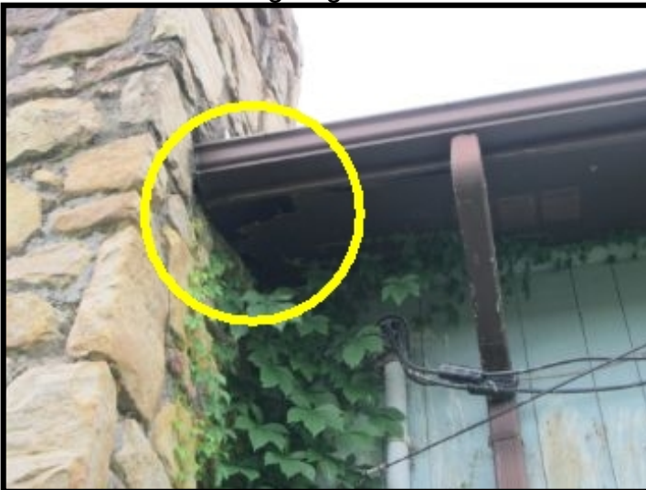
Soffit was rotted through at the side of the chimney penetration.
