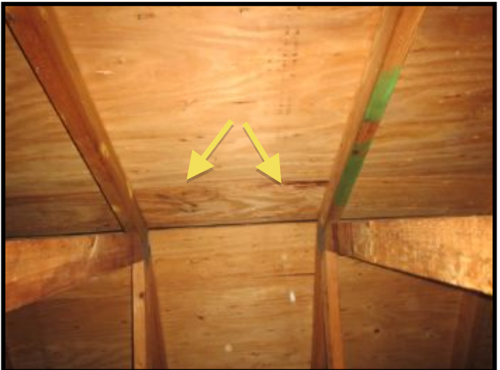
Water stains on decking in random areas in attic. water stains appear to be dry and could be from an old water leak from an older roof covering. Inspectors are unable to determine if stains are new or old. Inspector suggest keeping any water stains found anywhere through the structure a consideration and to monitor the stains during rains.
